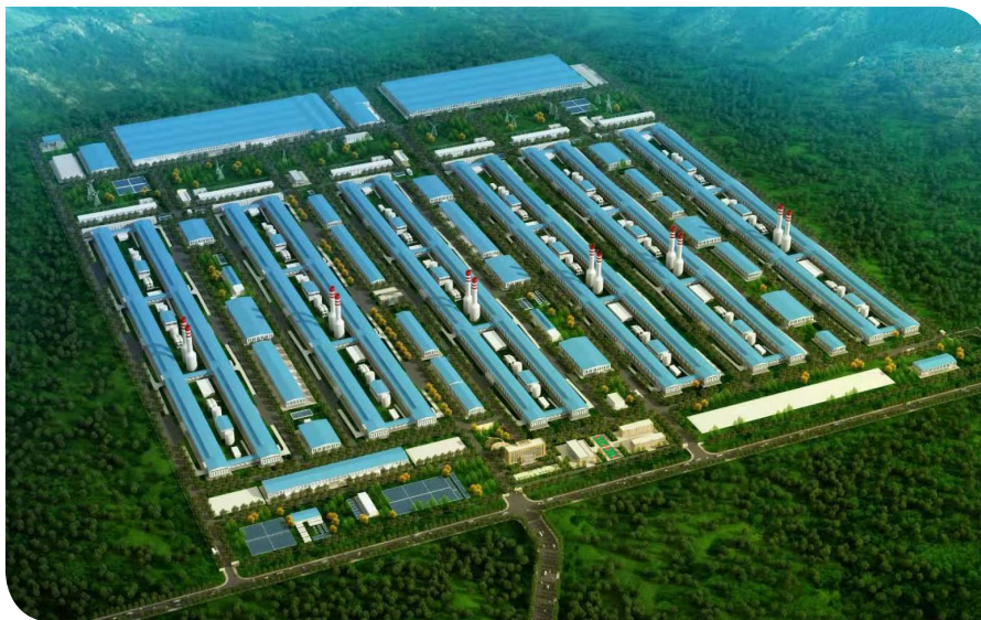
Yunnan green aluminium innovation industrial park
